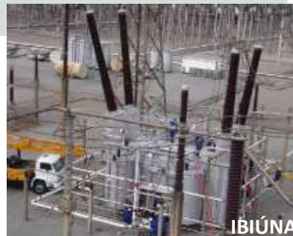
Trafos conversores HVDC 600 kV 300 MVA
