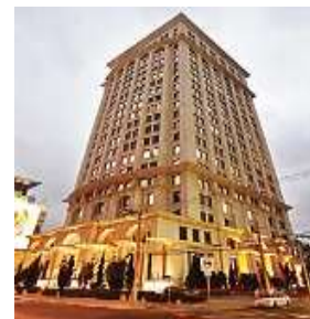
CHP Gas Natural – 3 MW Ed.Comercial, São Paulo
