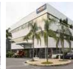
Gas Natural – 2 MW Hospital, Espírito Santo
