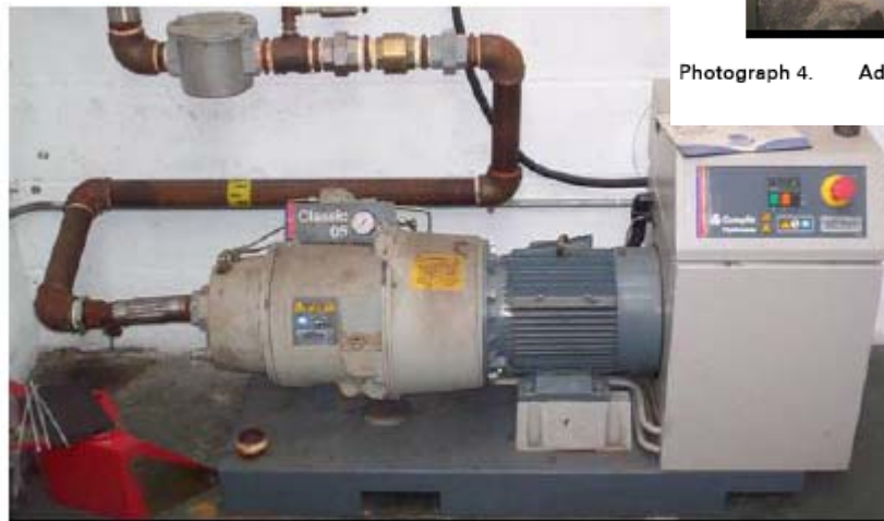
Photograph 3. Gas compressor model HV07
